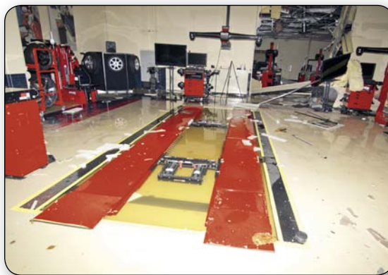
Gallons of water poured in from the damaged roof and sprinkler system, flooding the "PowerBay" and surrounding areas.
