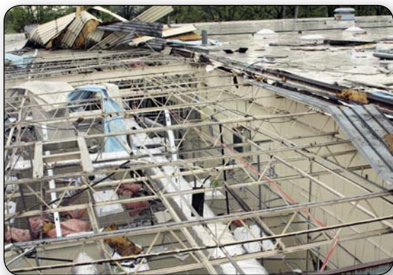
EF4 winds ripped a 5,000-square-foot hole in the roof structure, tore away 3,000-lb. AC units, and collapsed interior walls.
