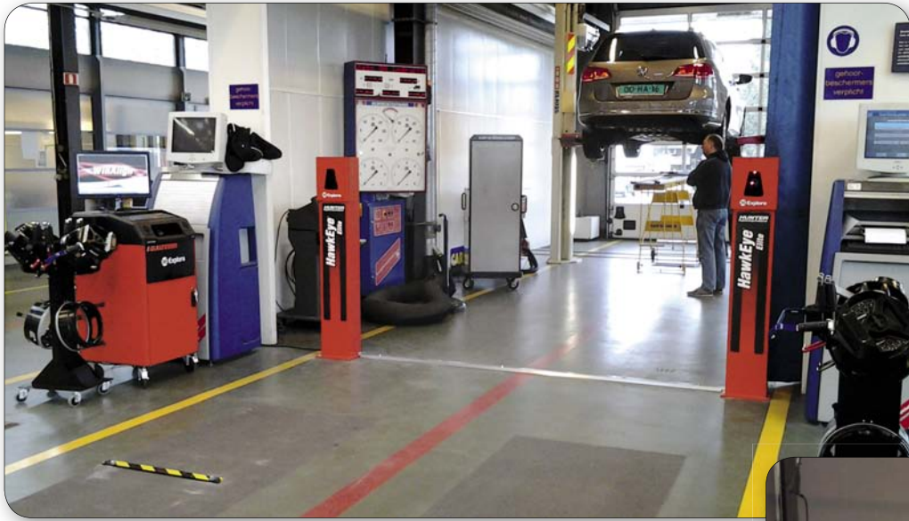
Above: A drive-thru Hunter Quick Check unit at an RDW inspection center in Zwijndrecht.
